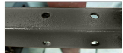
Dura-Coat OX applied over corrosion.
